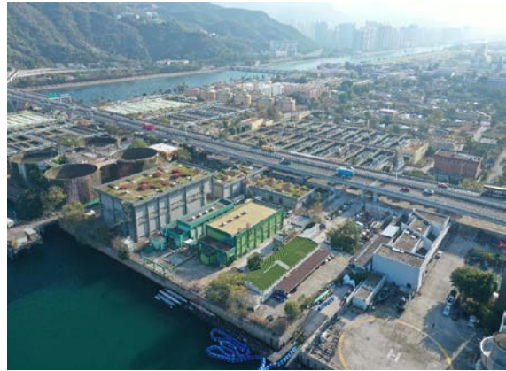
Figure 3.15: Sha Tin Sewage Treatment Works
