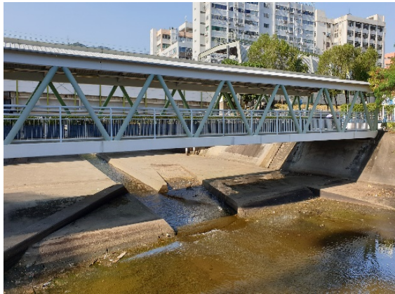
Figure 3.10: Shing Mun River section at Man Lai Court (upstream)
