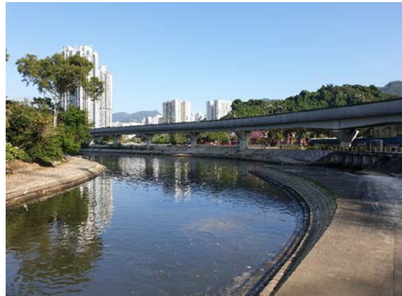
Figure 3.11: Shing Mun River section at Man Lai Court (downstream)
